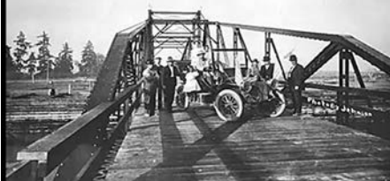
1909 Swing Bridge to Camano Island
