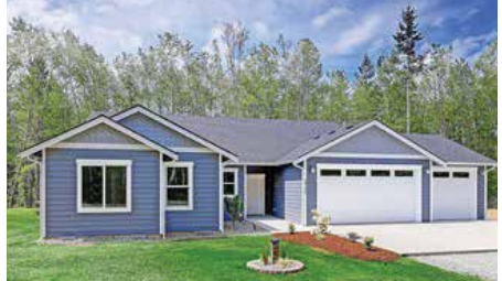
MOUNT VERNON $739,000 New construction in the Nookachamp Hills area with beautiful upscale finishes and wonderful community amenities. #1835235
