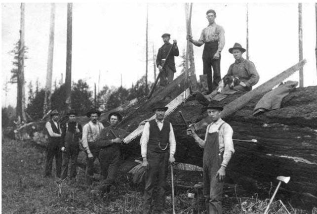
Loggers posed on downed timber with hand logging tools. ca. 1917. Photographer: Jensen, Auggie. Salvaging burned logs in Cedarhome area using crosscut saws, pike poles and peavey.
