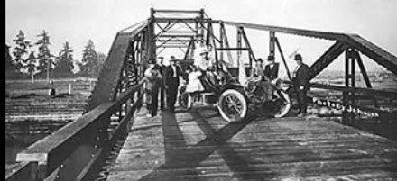
1909 Swing Bridge to Camano Island
