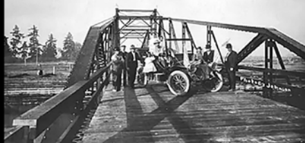
1909 Swing Bridge to Camano Island
