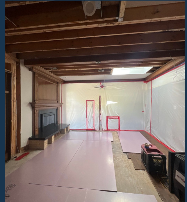
CONTAINMENT AND FLOOR PROTECTION
