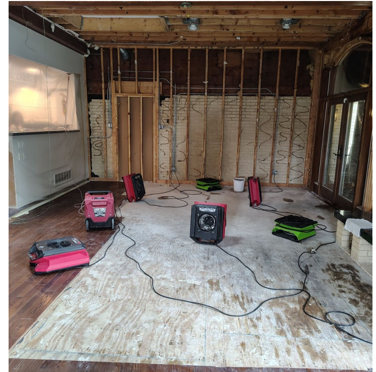
DRYING EQUIPMENT AND MONITORING
