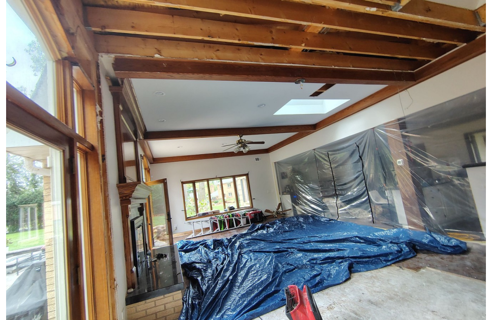
CONTROLLED INTERIOR DEMOLITION
