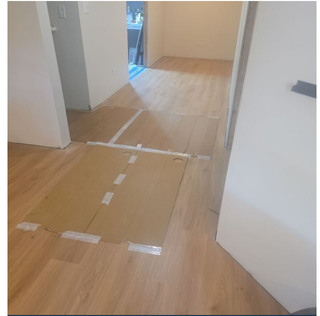
NEW FLOORING BEGINS
