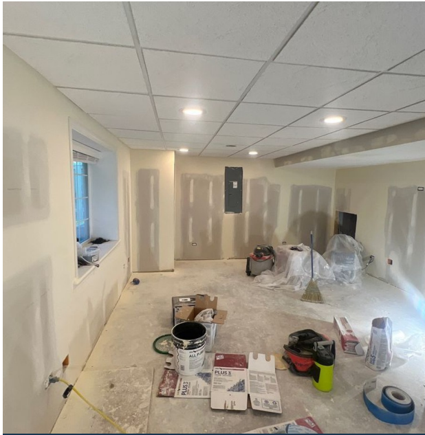
DRYWALL AND PAINT
