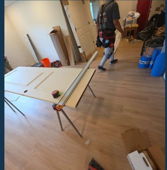
RECONSTRUCTION IN PROGRESS
