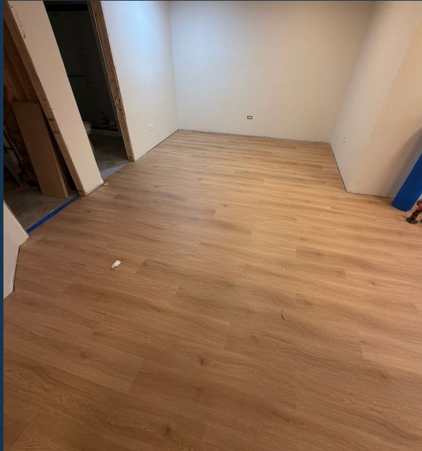
FINISHED AREAS RETURN
