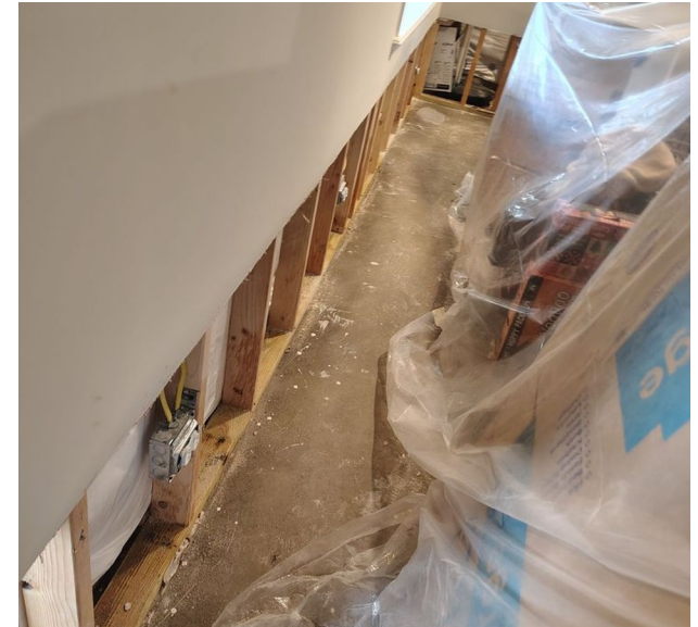
AFFECTED FINISHES REMOVED
