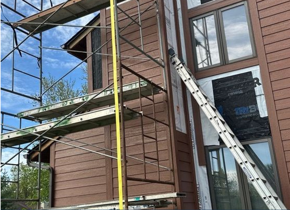
SIDING INSTALLATION IN PROGRESS
