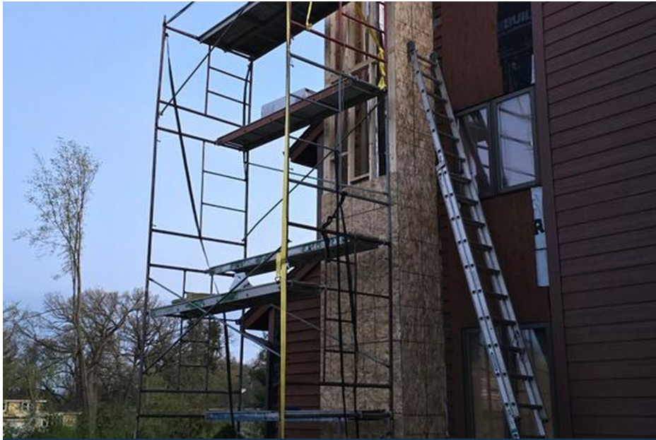
STRUCTURAL FRAMING AND SHEATHING
