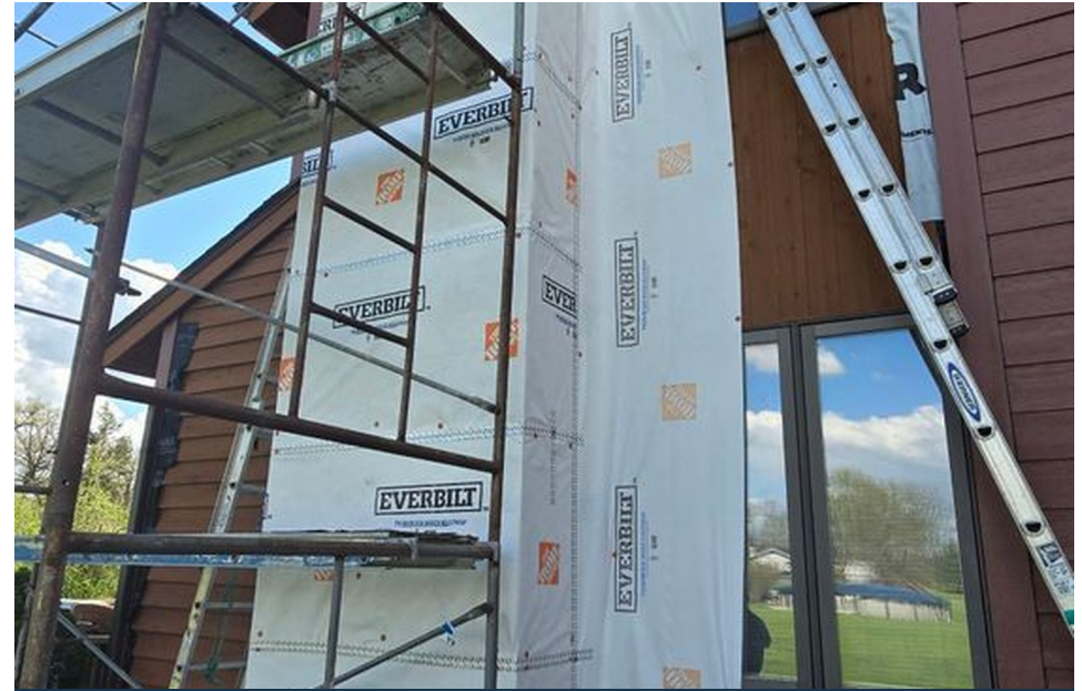
WEATHER-RESISTIVE BARRIER INSTALLED
