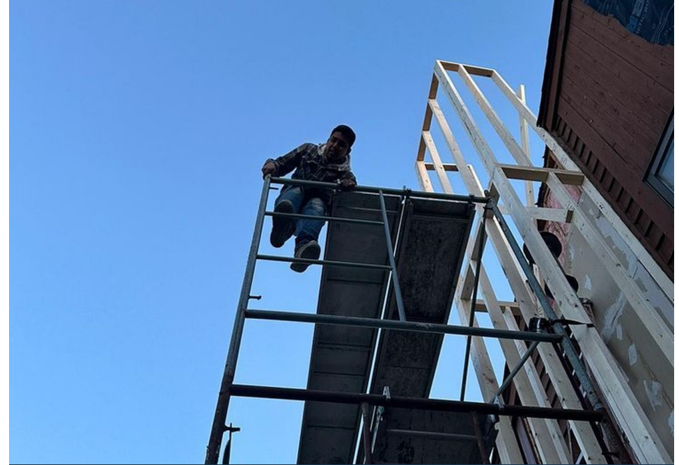
EXTERIOR FRAMING REBUILT
