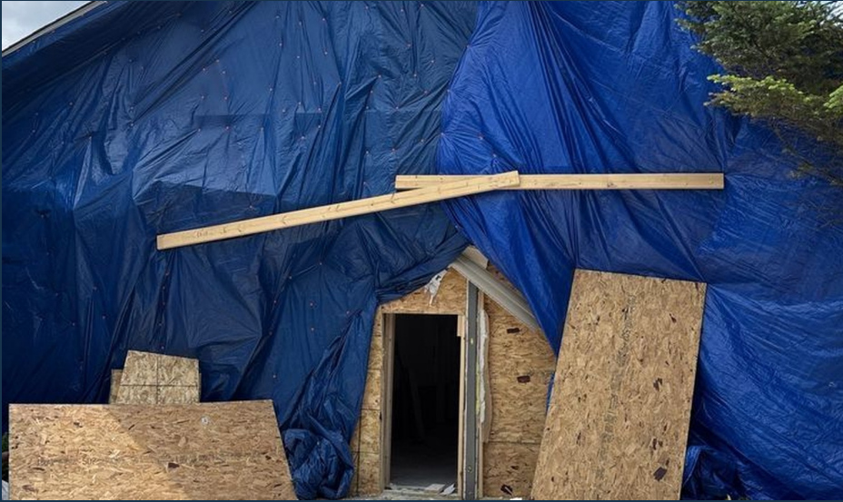
TEMPORARY WEATHER PROTECTION
