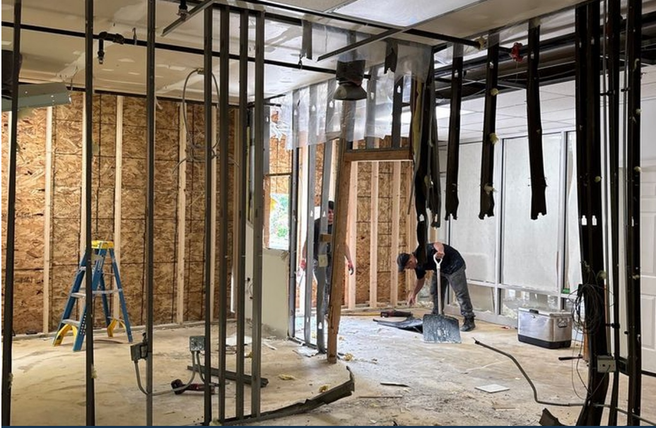
CONTROLLED ACCESS AND DEMOLITION
