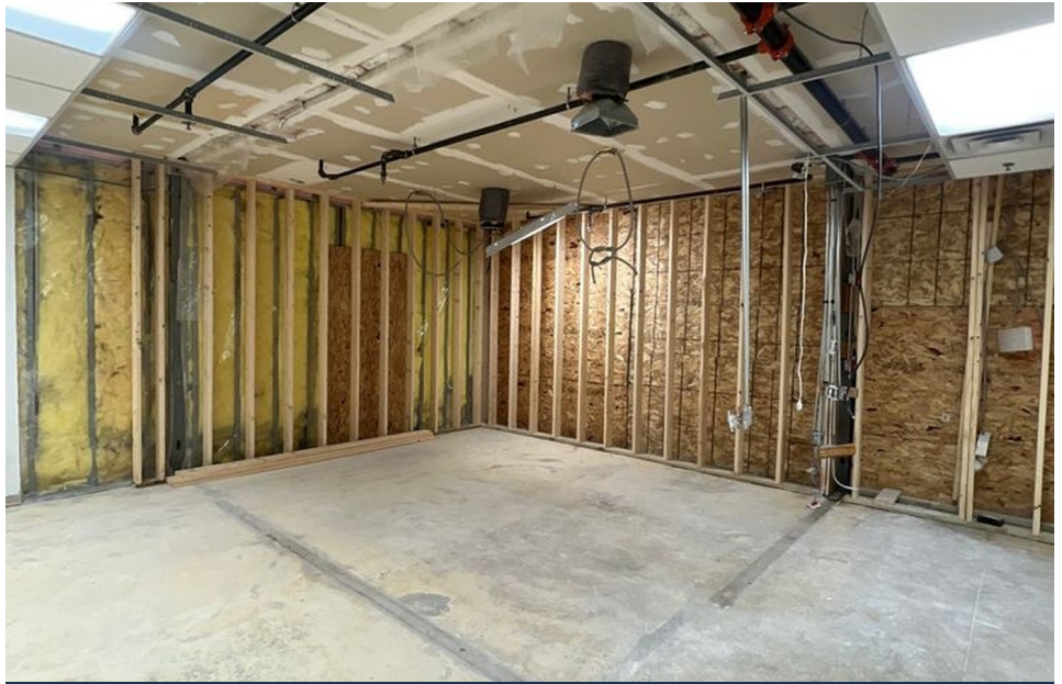
FRAMING OPENED AND REPAIR AREAS DEFINED
