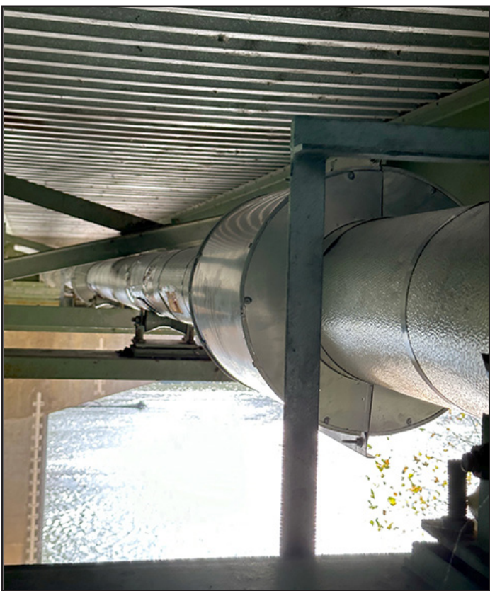
Shown above is the 750-foot wastewater line under White River, East Fork Bridge.
