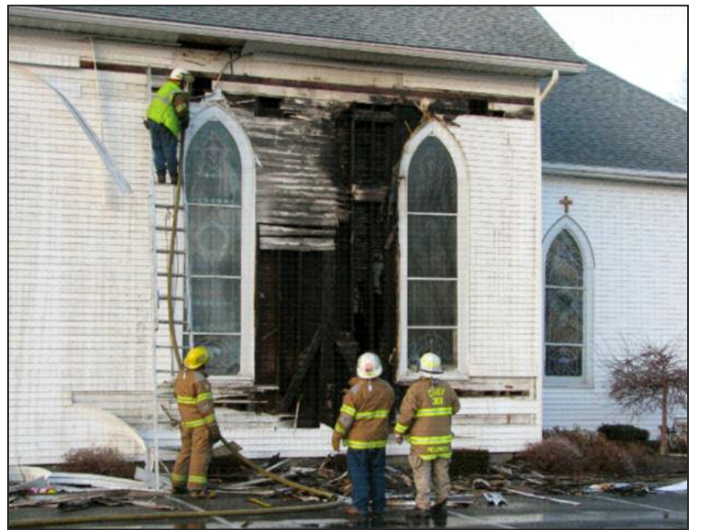
St. Joseph Church almost repaired -Photo above provided
