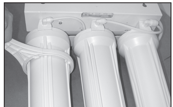
Figure 11 - Using sump wrench to change filter cartridges
