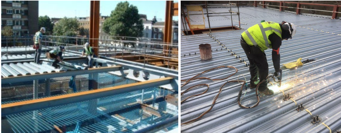
The installation of metal decking and through deck stud welding
