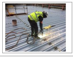
Shear studs are required to transfer force between the steel section and the concrete slab. The studs are welded to the beam, normally through the deck sheet. This enables the concrete slab to act like a large top flange to the composite beam when the concrete has hardened and creates a stronger section to support the loadings applied to the finished slab.
