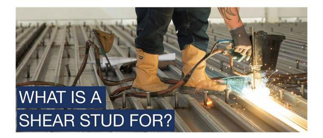
The increased performance of composite beams, in stiffness and bending resistance, allows the construction of longer spans and shallower floors when compared to non-composite methods. This could allow smaller storey heights, more floors for the same building height, more flexible column free areas and increased opportunities for services.
