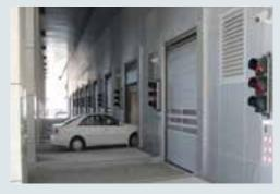
Cars enter through openings with high speed roll-up doors - traffic lights signal when it's safe to enter
