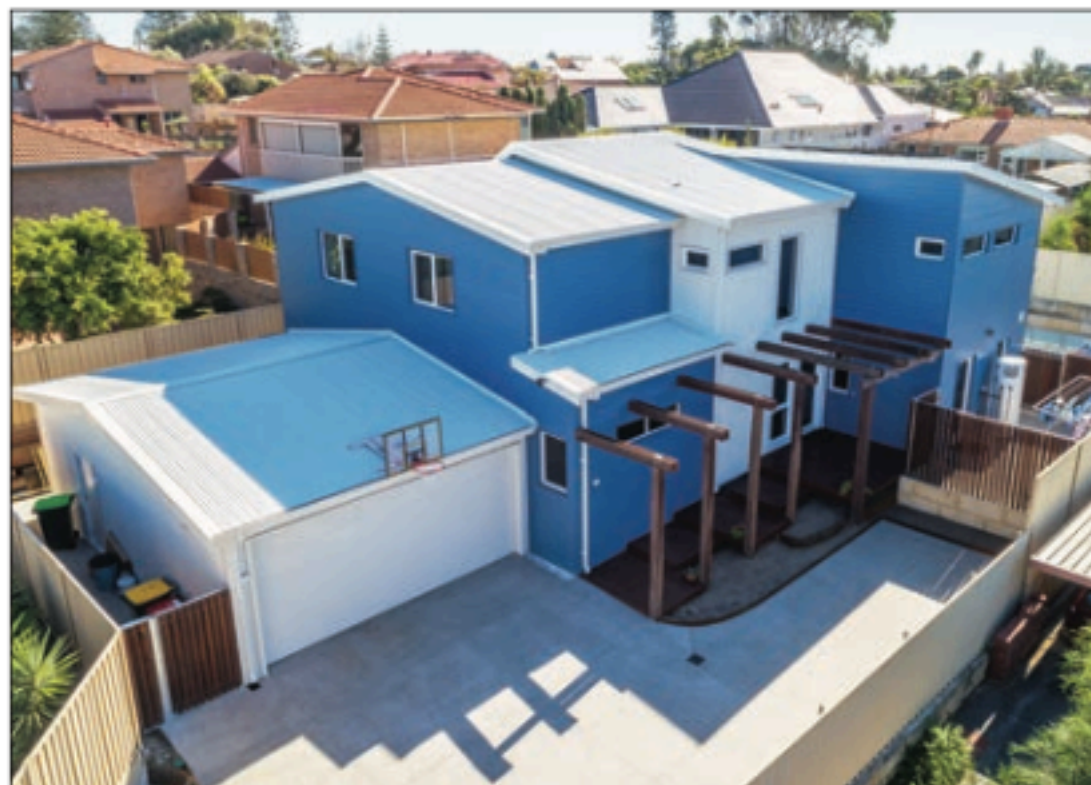
• The first 'passive house plus' in WA (above). The owners spent the energy bill savings on wine (left).
