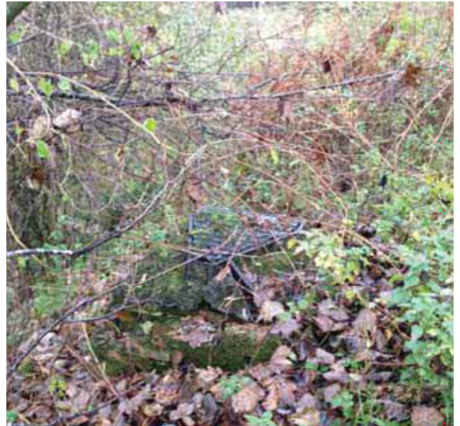
19) Drainage manhole in northeastern site area
