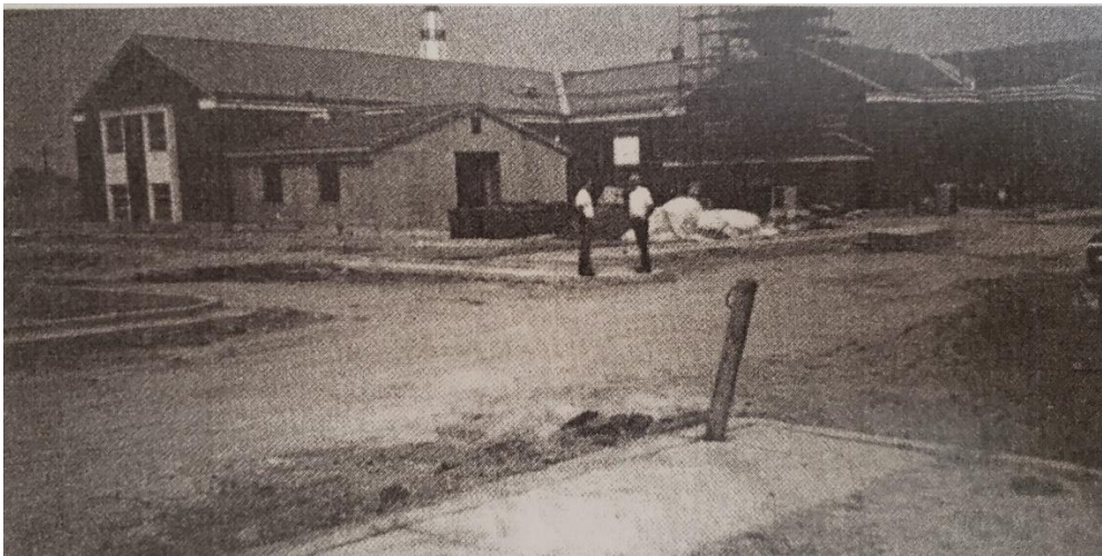
Remodeling of Hawthorne & Quinn Building
