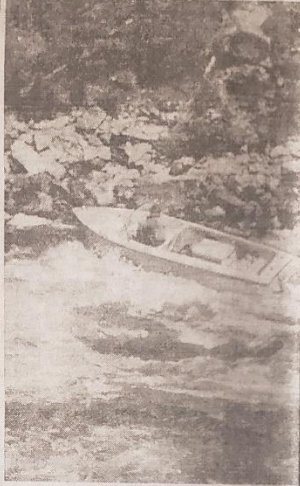
ONCE IN RAPID, DRIVER PICKS SLICK OF RIVER ... "Propelled" by turbine—makes water-jet stream
