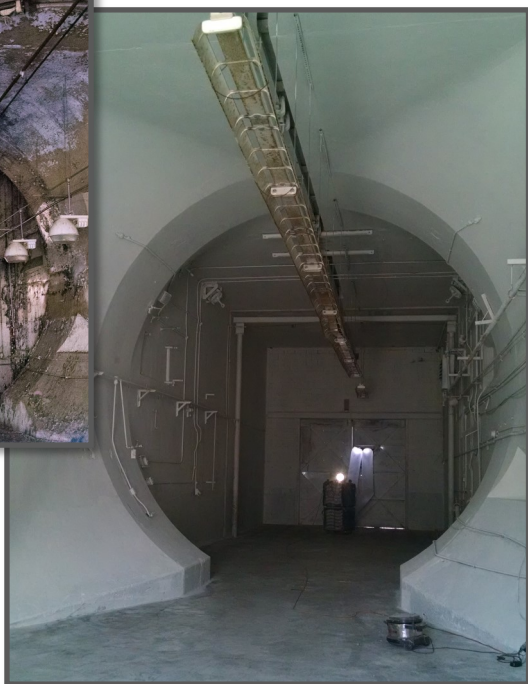
Lead-based paint stabilization before (above) and after (right) abatement.
