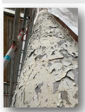
LEFT: Close-up of column before lead-based paint stabilization process
