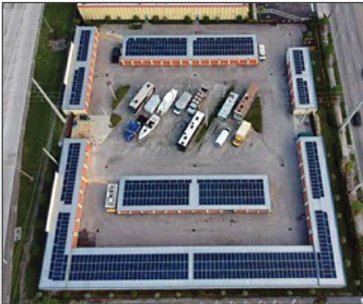
150kW Solar PV installation on Mini Storage facility, Miami, FL
