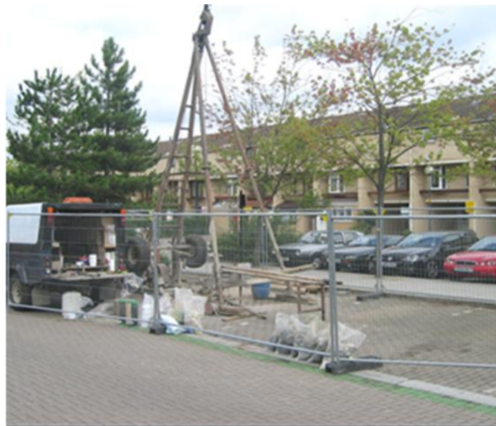
Example of site protection
