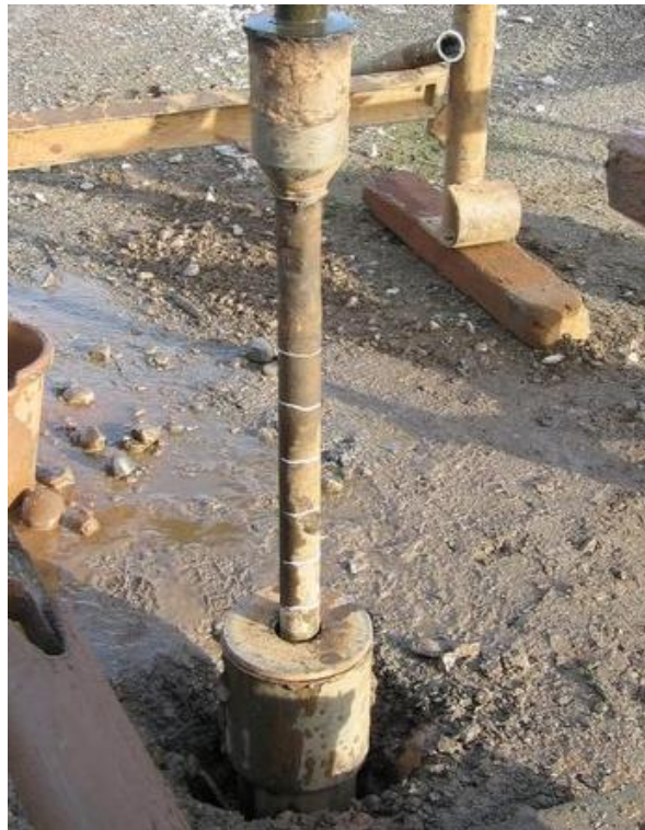
SPT rods marked up for a test also showing the centralising collar
