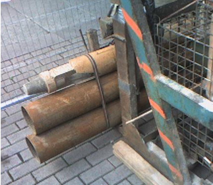
Casing and tools being used as a counterbalance
