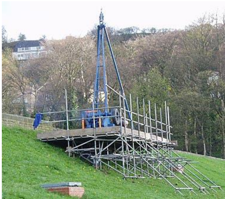
Cable Percussion rig set up on a scaffold platform
