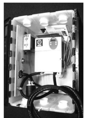
VFD mounted in box
