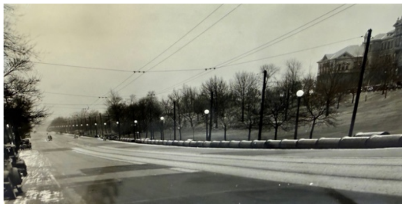
(Photo from Cincinnati Historical Society-Clifton Archives) Clifton Avenue Looking North, 1906 Overhead Streetcar electric wires Lined with globe-topped, Boulevard style streetlamps
