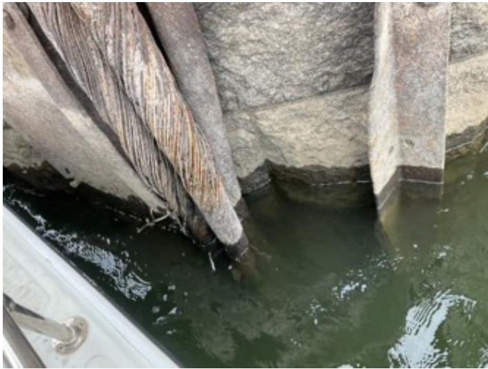
(F) NW Broadway Bridge cables. WR 7. August 2022, Portland, Oregon.
