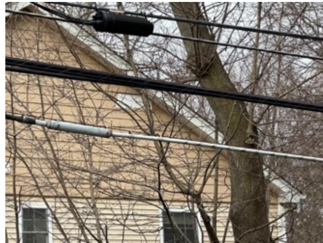
(C) Exposed bare lead splice box and lead cable. January 2023. Highland Falls, New York.
