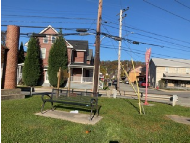
(A) Park bench near exposed lead sheathed cables and splice boxes. October 2022. Natrona, Pennsylvania.
