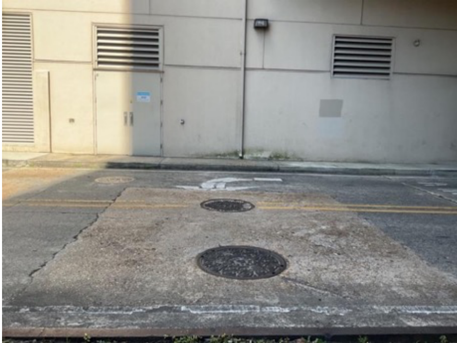
(I) New Orleans, LA. MISS 2.1 with Bell Systems manholes, vault, and Utility Building. This is a likely hub and splice area for cables, both old and new. June 2022.
