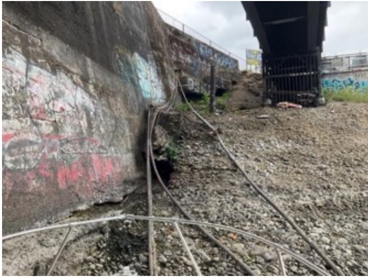
(E) North Steel Bridge cables. WR 6. August 2022, Portland, Oregon.
