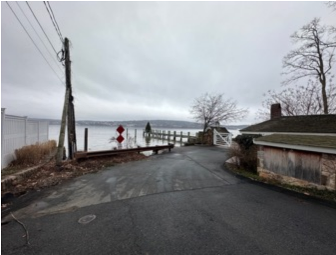
(H) Abandoned 5" lead sheathed cable along the Hudson River. January 2023, Palisades, New York.
