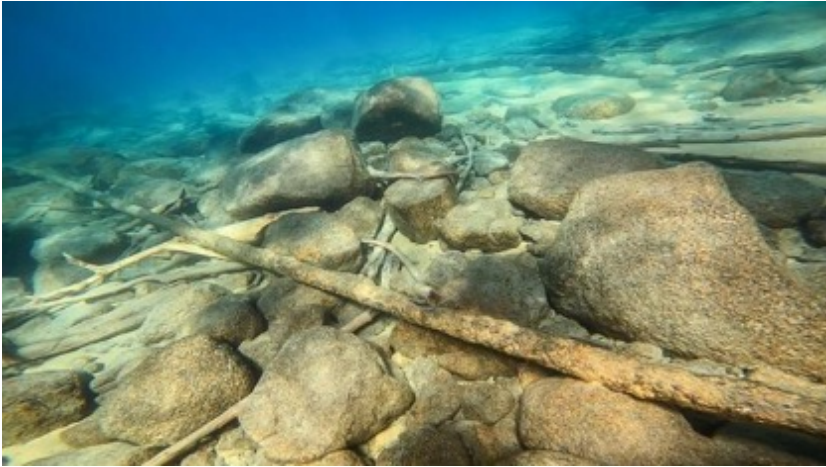
(D) Lead sheathed cable laying among boulders on the lake bottom. April/March 2022. Lake Tahoe, California.
