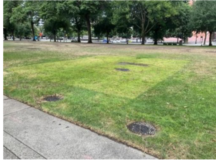
(C) Five Bell Systems manholes with vault. WR 2.2. August 2022, Portland, Oregon.
