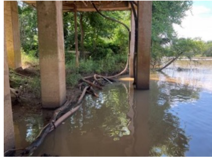
(E) Rd. 320 southeast of New Iberia, LA. Cluster of lead sheathed cables under the Oliver Bridge. BT 17.1. June 2022, New Iberia, Louisiana.
