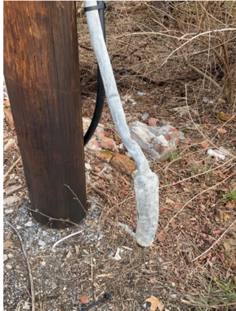
(G) Damaged lead cable and splice box at the base of an old telephone pole. Point of Interest: New Windsor 1. January 2023, New Windsor, New York.
