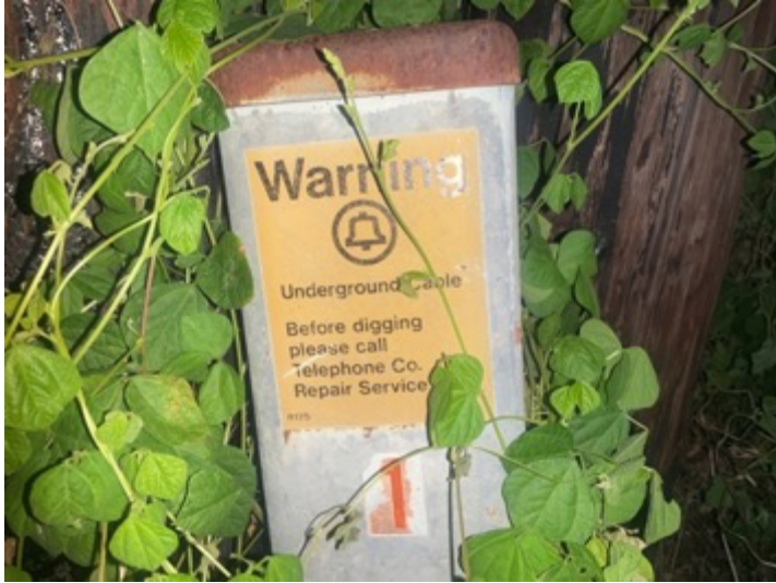
(A) Bell Systems sign for underground Telephone Cables. BL 2.1. Labadieville, Louisiana. June 2022.
