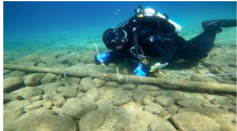
(C) Diver marking locations of damage during a survey in April/March 2022, Lake Tahoe, California.
