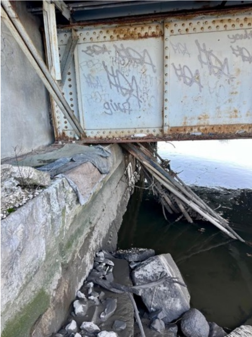
(H) Evidence of homeless sleeping next to these cables along the Passaic River. Passaic 2. January 2023, Harrison/University Heights, New Jersey.
