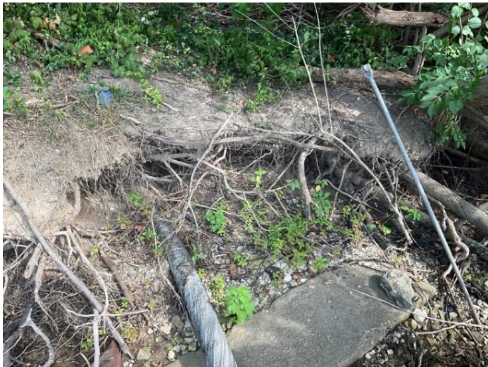
(D) Lead sheathed cables from (C) continuing past the tree line. They are buried in the ground and run up the hill to a Bell Systems manhole. DR 1. July 2022, Trenton, MI.
