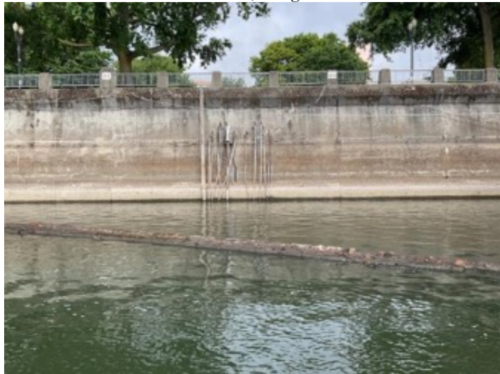
(B) Eleven cables near Maritime Museum and Waterfront Park. WR 2.2. August 2022, Portland, Oregon.
