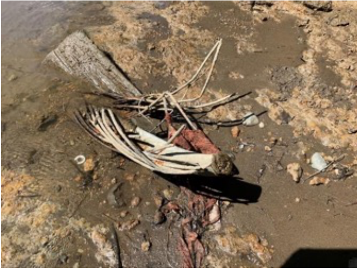
(A) Abandoned lead sheathed cable near Ross Island. WR 1. August 2022, Portland, Oregon.
