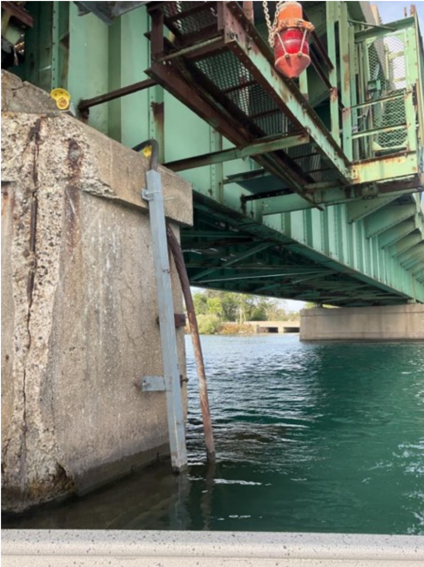
(E) Lead sheathed cable along the Grosse Ile Parkway Bridge. The cable runs through the concrete and is cut just above the ledge. DR 2. Grosse Ile Township, MI
