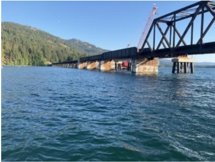
(A) Lake Pend Oreille, ID Railroad Bridge. August 2022.
