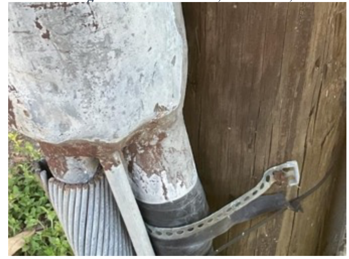
(F) Up close photo of bare lead sheathed cables coming from the bottom of a lead splice box (upper left corner of photo). BT 24.1. June 2022, St. Martinville, Louisiana.
