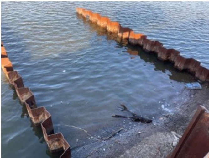
(B) Cable landing area covered with concrete. Area is below the sign in (D). January 2023, West Side, New Jersey.
