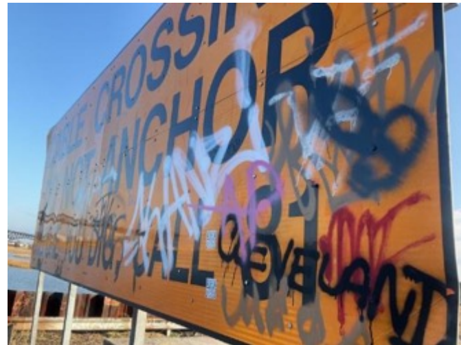
(D) Cable Crossing Sign. January 2023, West Side, New Jersey.
