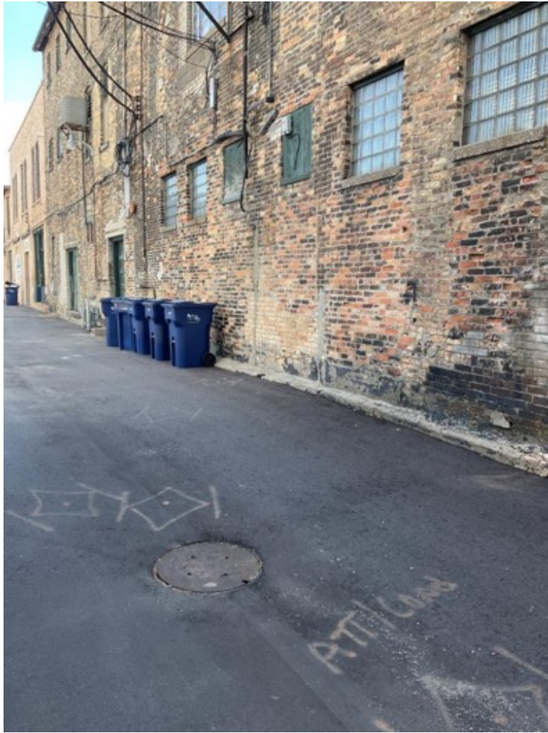
(A) Paint Markings indicating an AT&T service corridor. The lead sheathed test line follows these markings along the brick building shown above. LH 2.2. July 2022, Bay City, MI.
