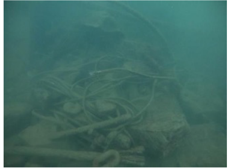
(F) Lead sheathed cables abandoned and coiled below the surface. Site LP 4.1. August 2022, Lake Pend Oreille, ID.
