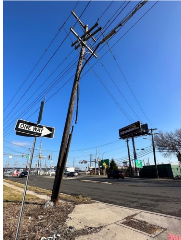
(B) Overhead cut, lead sheathed cables in the South Kearny area. There are two cables that run approximately 0.4 miles. South Kearny End A. January 2023, Kearny, New Jersey.
