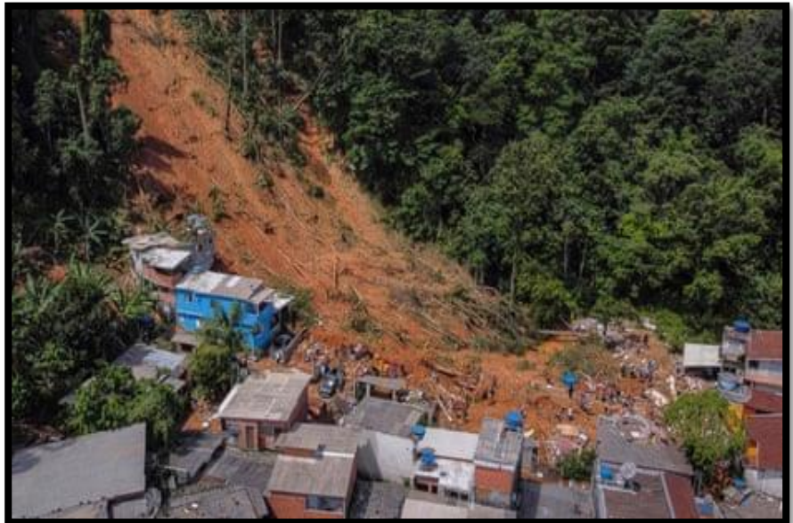
Figure 2: The destruction left after torrential rain in the state of São Paulo- Image by Fernando Marron
