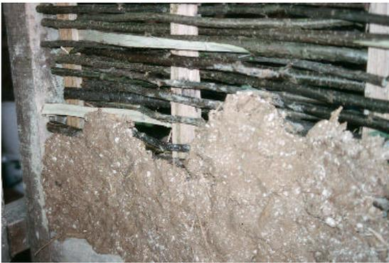
Figure 6. Wattle and Daub Wall Construction
