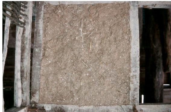
Figure 7. Wattle and Daub Wall Construction
