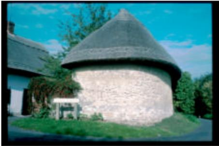
Figure 1. Cob Walling Construction in England
