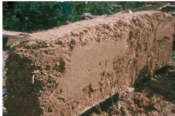
Figure 3. Building a Cob Wall
