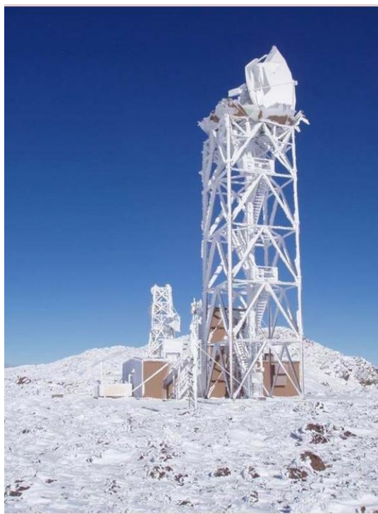
Figure 87: NWS Reno Radar Damage from Wind, December 2008 146
