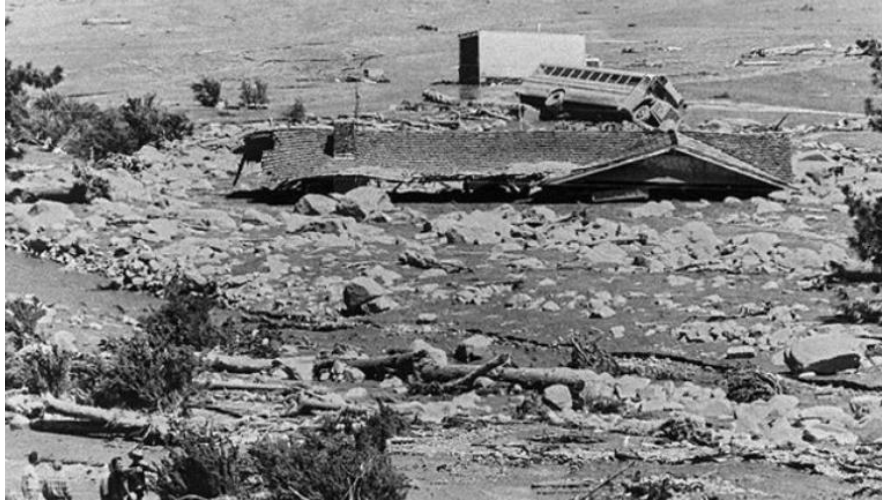
Figure 20: Photo of the Slide Mountain Landslide, May 30, 1983 44
