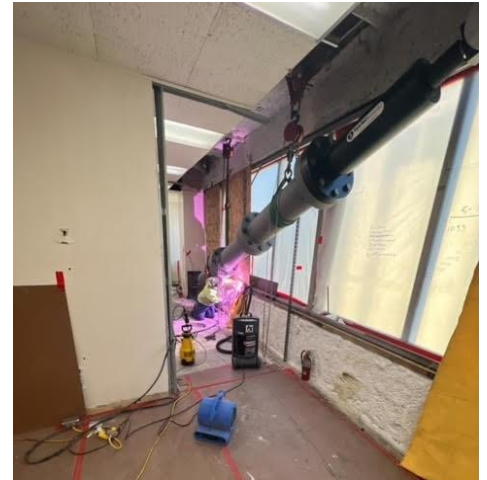
Figure 73: Seismic Retrofitting in the City of Reno City Hall
