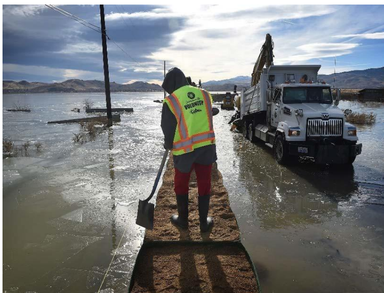
Figure 100: Flood Barriers Being Set Up on the Edge of Swan Lake by Washoe County 168
