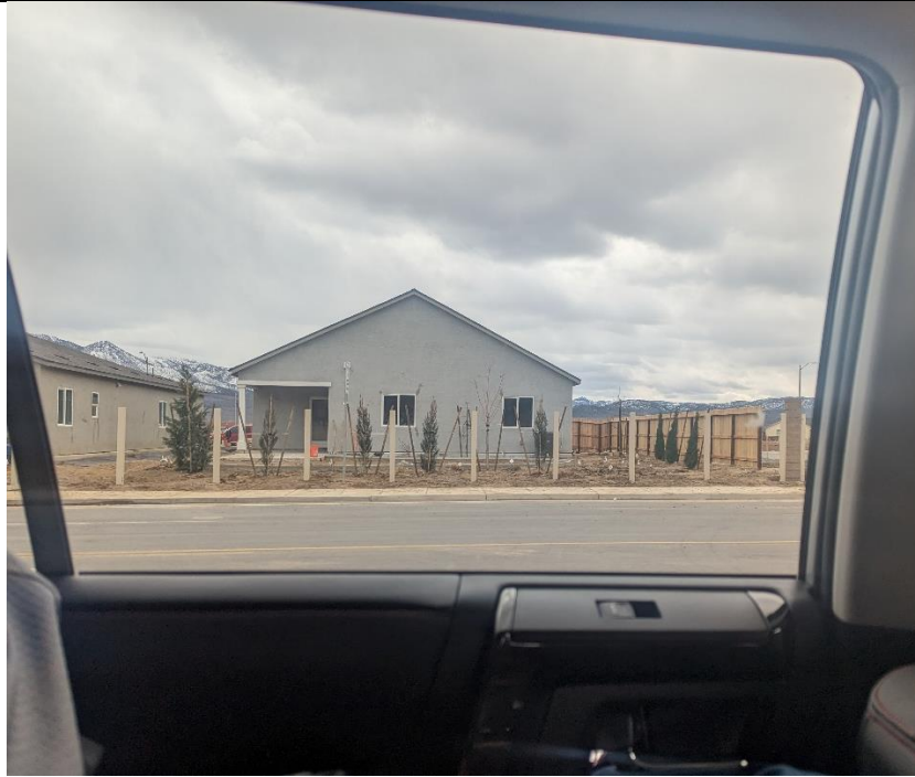
Photo 3. Image of the Traditions Development in progress where sampling has not followed the finalized 2018 LTSRP
