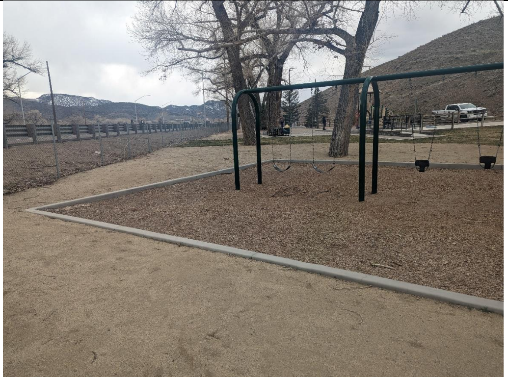
Photo 5. Image of the Union Park playground and the swing supports that go into the cap under the playground.
