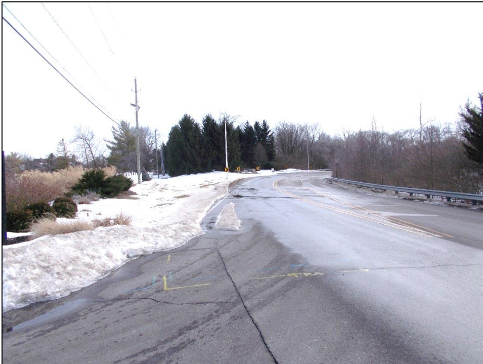
Looking south along Westfield Boulevard from the site entrance.
