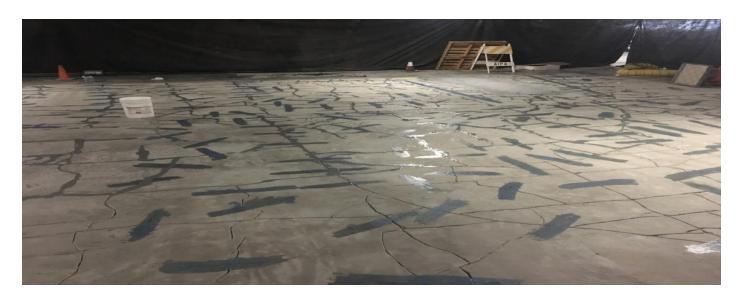
StitchDog<sup>TM</sup> Carbon Fiber Grid Stitches being installed after cracks were prepped, cleared of loose concrete and area cleaned and vacuumed. Saw cuts are made perpendicular to cracks using a standard circular saw with concrete blade. Because of the failure was so extensive, some of the StitchDog<sup>TM</sup> CFGS are covering multiple crack lines.
