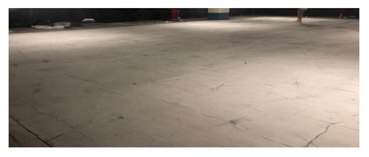
After all of the cracks were repaired with the StitchDog<sup>TM</sup> CFGS System, the test area was allowed to cure for 24-hours to ensure no degassing of the epoxy would affect the overlay system. This image shows the surfaced prepped with a grinder to a profile necessary for the park deck coating system.
