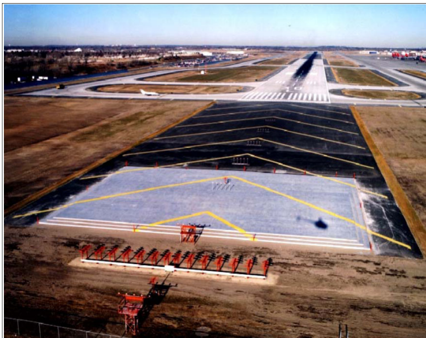
FIG 2-3-42 Engineered Materials Arresting System (EMAS)
