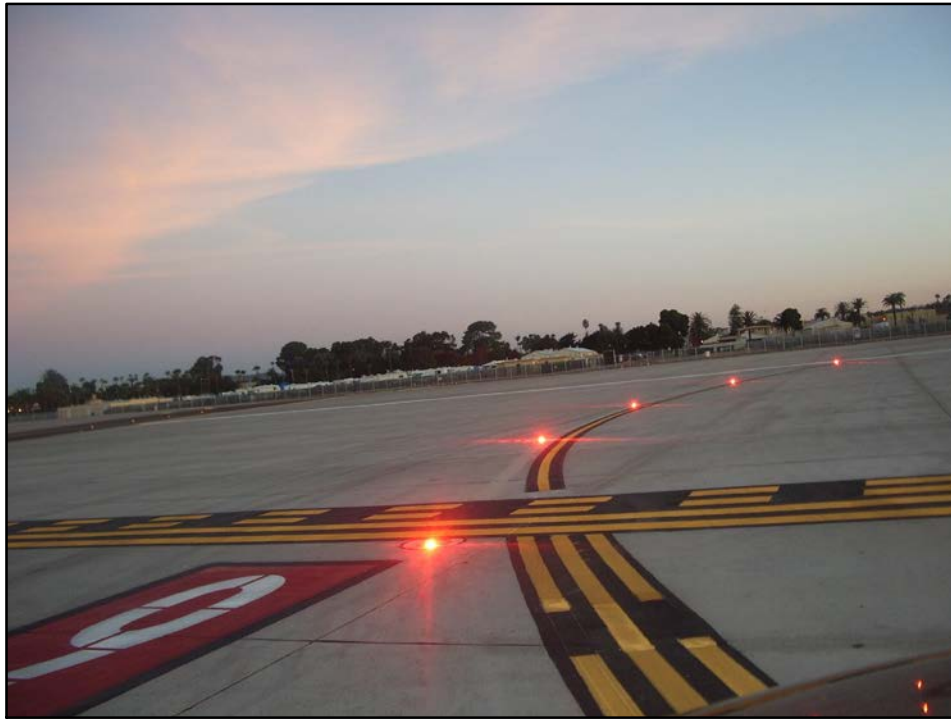
FIG 2-1-10 Runway Entrance Lights
