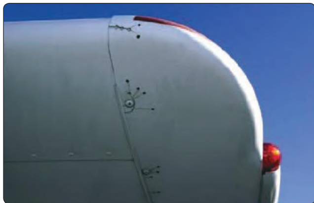
Figure 2-8. Cracks radiating from screw holes that have been stop-drilled to prevent crack progression.
