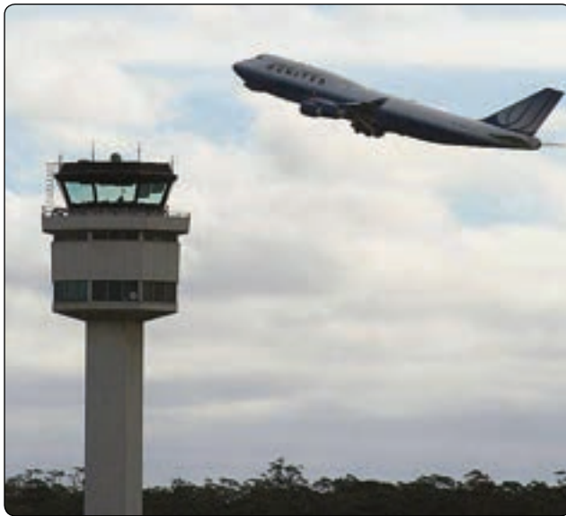
Figure 5-7. National airspace voice switch (NVS) will replace existing voice switching systems with single air/ground and ground/ground voice communication systems.
