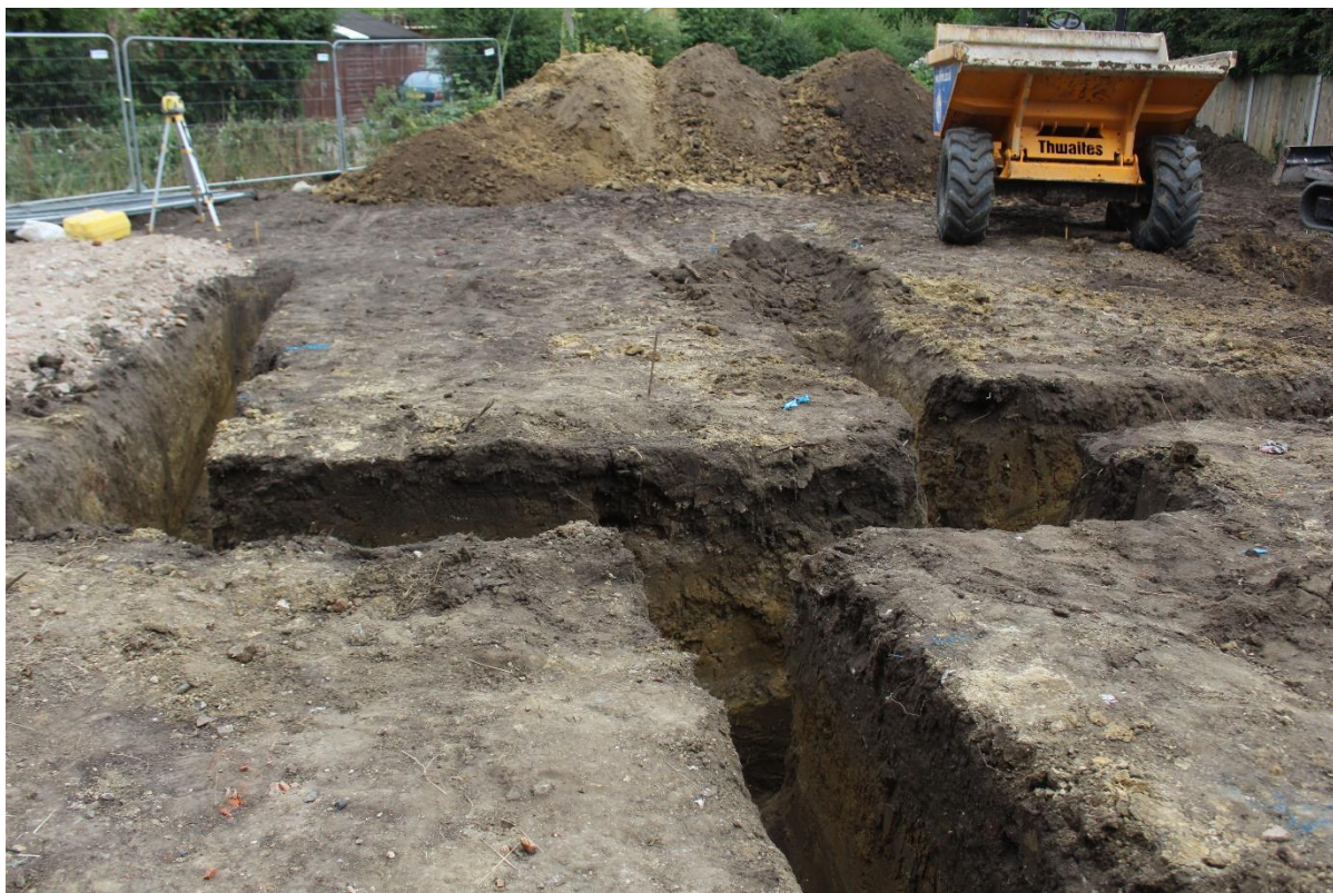
Plate 3 General view of trenches facing east-south-east
