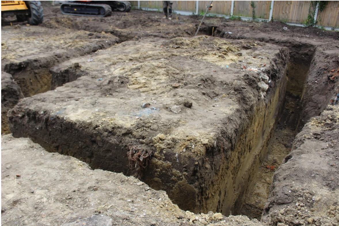
Plate 1 General view of trenches, facing south
