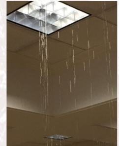
Fellowship Hall Damage
