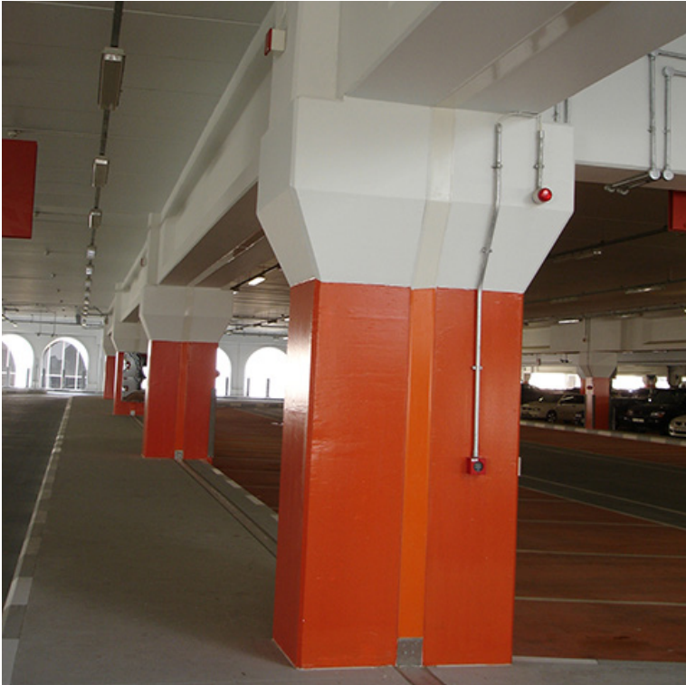
CJ - Parking Mall of the Emirates - Dubai - EMIRATOS ÁRABES UNIDOS
