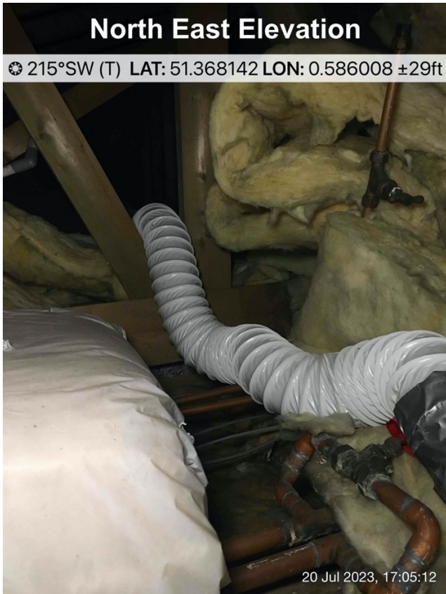
Ducting not extended to full length.
