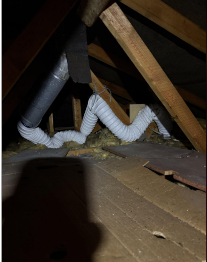
Incorrect vent type with poor external finish
