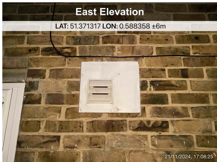
Incorrect vent type with poor external finish
