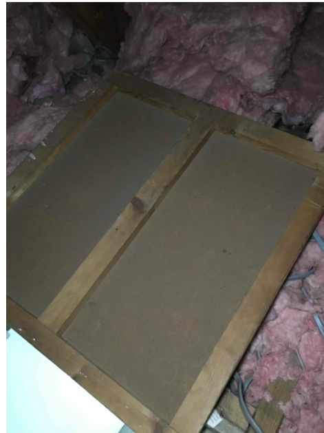
Layer of wool not consistent with loft insulation
