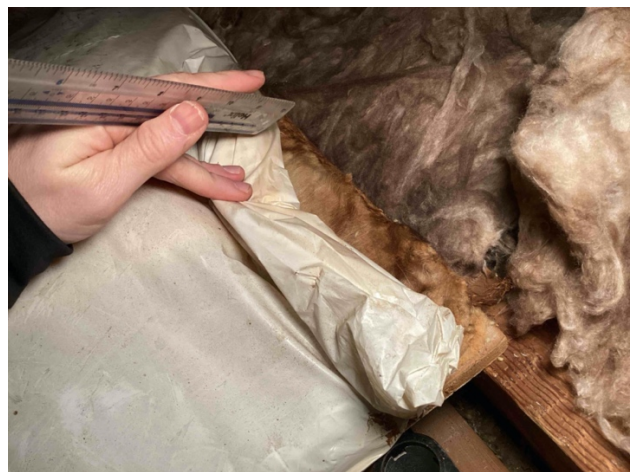
Layer of wool not consistent with loft insulation
