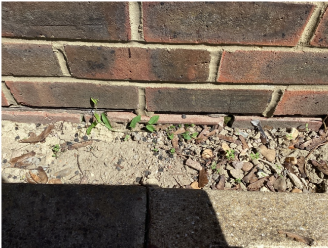
Airbricks blocked by ground level:
