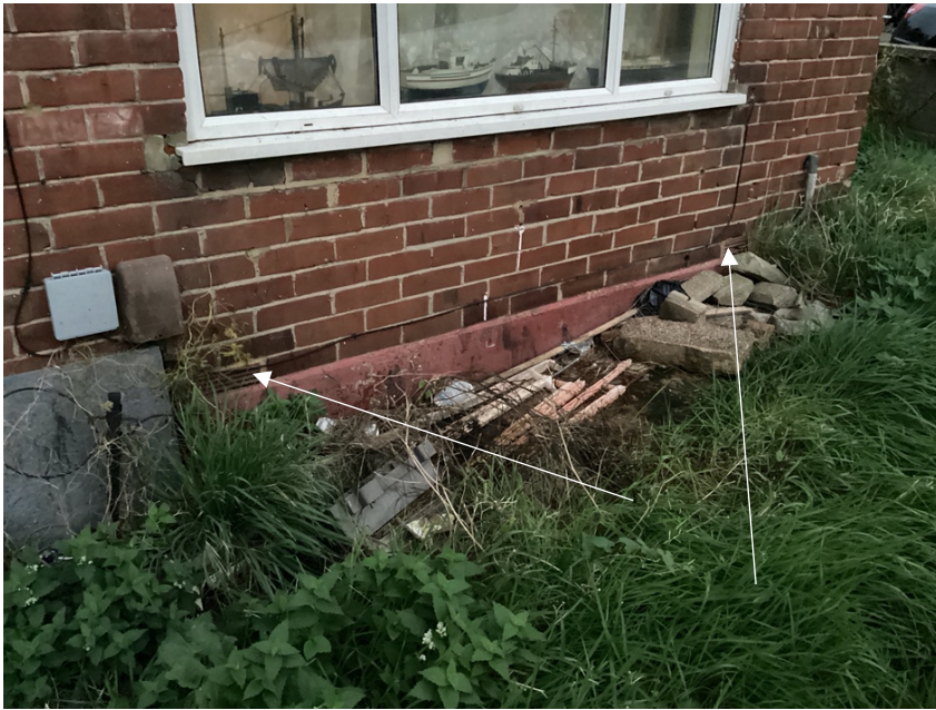
Airbricks blocked by ground level:
