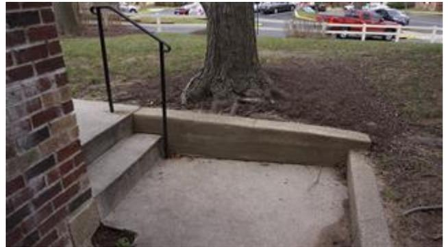
The brick retaining walls are primarily located at the below-grade accessways to the laundry rooms and storage rooms at either end of each of 12 buildings and at one end of three buildings. The condition of these walls varies from good to poor, with the primary deficiencies being loose and missing mortar, loose and missing brickwork, loose and deteriorating brickwork at metal railing bases, through-wall cracking, and deterioration of surface parging.
