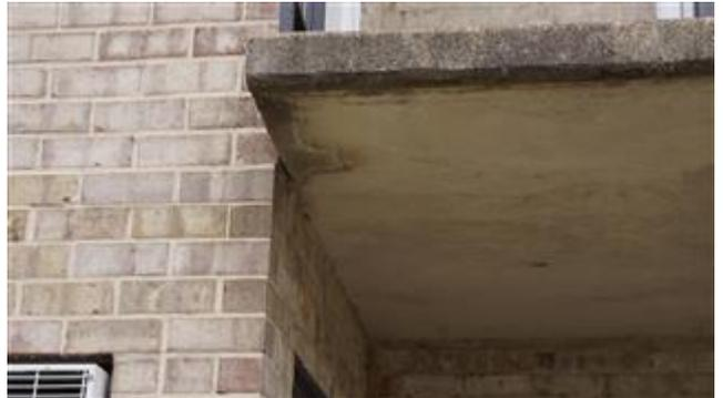
We noted no major defects which appear to be significant, although cracking in the concrete decks near support structures, cracks in supporting brick masonry, and spalling of brick at balcony bearing locations is noted. These defects should be closely monitored to determine if any of these conditions worsen over time.
