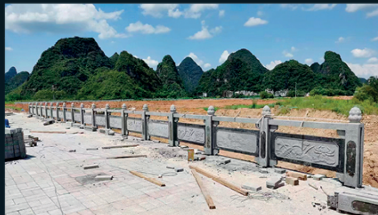
sesame black granite railing installation
