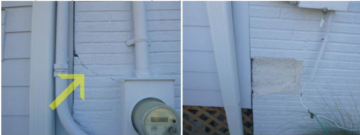
13. Damaged/missing stucco noted on the right side yard.
