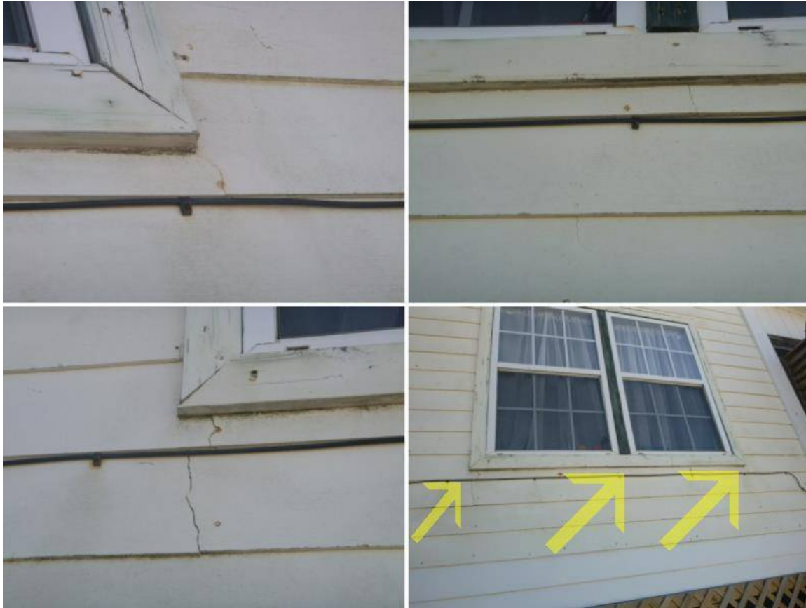
10. Some cracking/damage noted on the right side yard stucco wall at window. Recommend sealing cracks as needed.
