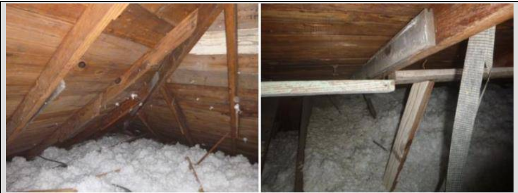
Some hip ridges appears to have slight sags from missing or damaged bracing. Recommend further evaluations by a licensed contractor.
