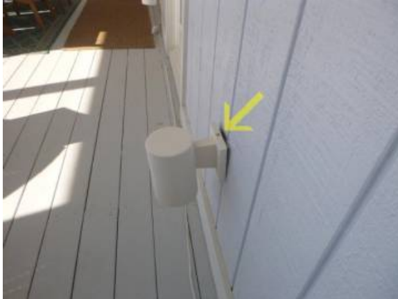
50. Loose light fixture noted at the rear screen porch.
