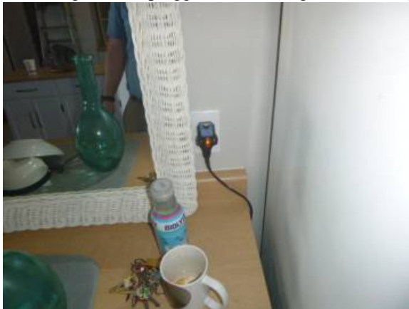
51. Refrigerator is plugged into a non-grounded receptacle. Shock hazard exist.
