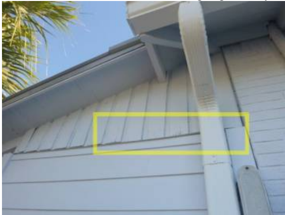
12. Wood rot noted on exterior siding: right side yard front upper siding.
