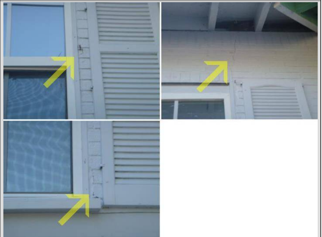
Some cracking/damage noted on the right side yard stucco wall at window. Recommend sealing cracks as needed.
