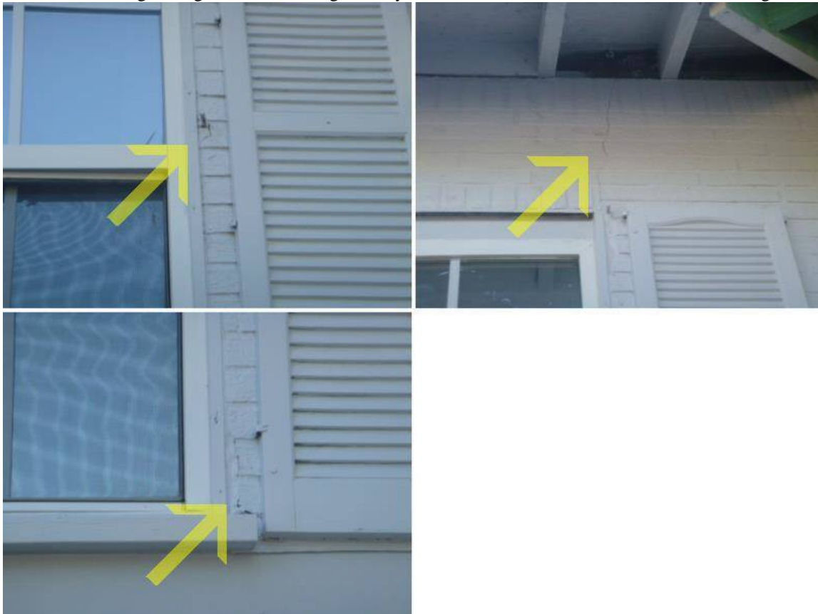
10. Some cracking/damage noted on the right side yard stucco wall at window. Recommend sealing cracks as needed.
