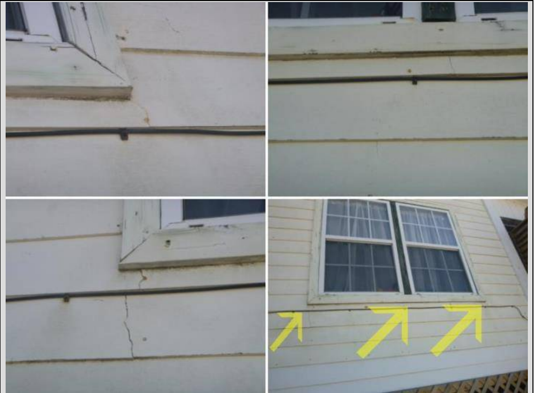
Cracked/damaged siding noted on the right side yard siding, recommend repairs to prevent further damage/deterioration.
