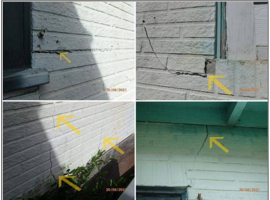
Various areas of cracking / damage to stucco at the East side near the front NE corner.
