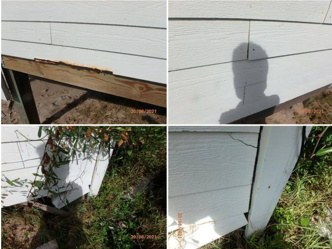
15. Various areas of damage noted to the siding on the East side of the house.
