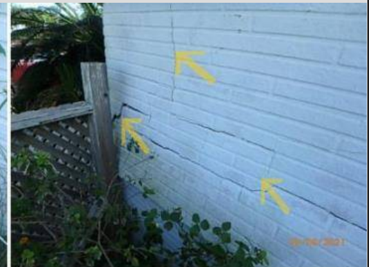
Significant cracking / damage to stucco from settlement at the West side near the front NW corner.
