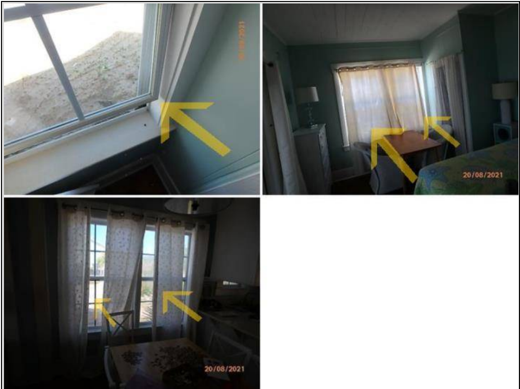
Windows will not stay open in the following locations: master bedroom windows, dining area windows. Windows do not stay in track properly.
