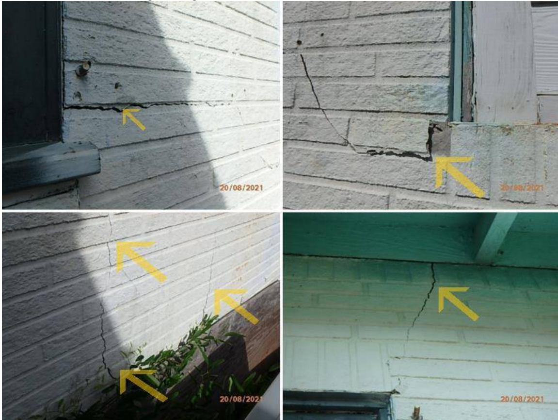
10. Various areas of cracking / damage to stucco at the East side near the front NE corner.
