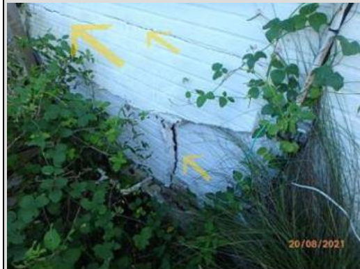
Significant cracking / damage to stucco from settlement at the West side near the front NW corner.
