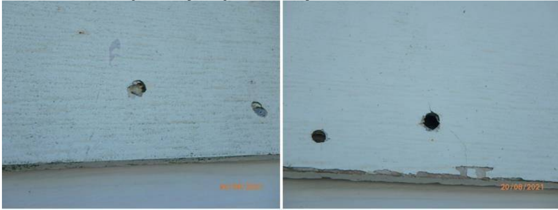
14. Various holes / damage in the lap siding material from pulled out nails.
