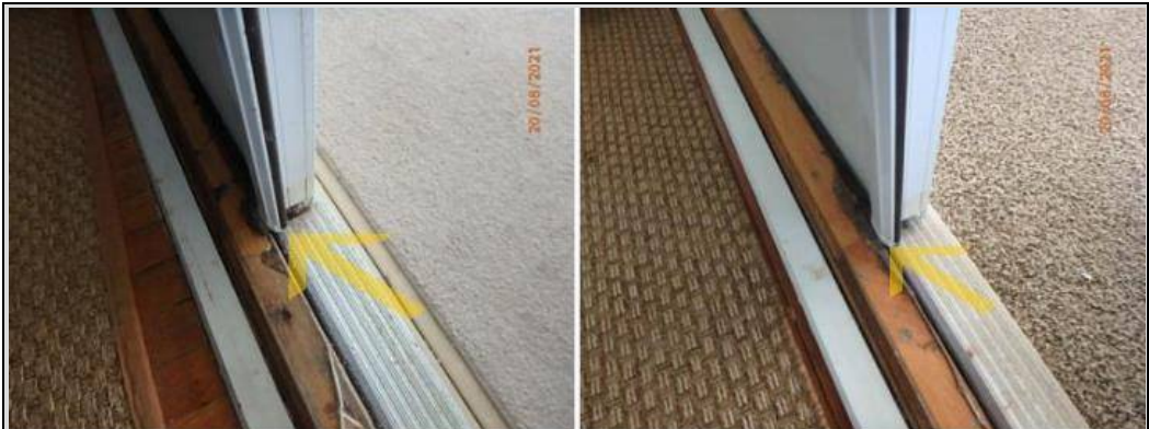
The middle french door and the master bedroom french door bottom set pins will not properly engaged due to the bottom of the doors being in conflict with the threshold. Adjustment is needed.
