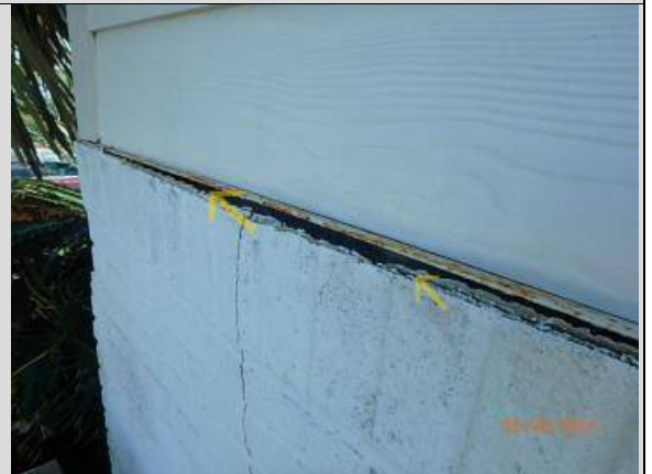
Significant cracking / damage to stucco from settlement at the West side near the front NW corner.
