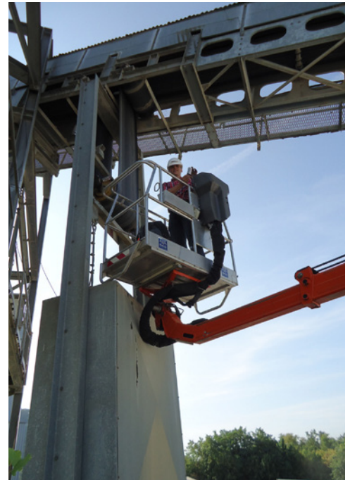
Thanks to simalube lubrication points at unreachable heights are also constantly supplied with lubricant.
