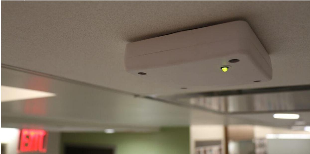
*The gunshot detection system works both outside and indoors with sensors placed in critical areas on each floor of the buildings and a breezeway connecting the two campuses. The unobtrusive sensors resemble a Wi-Fi extender.*
