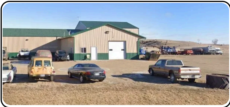
RYAN'S REPAIR (MONTROSE, SD)
