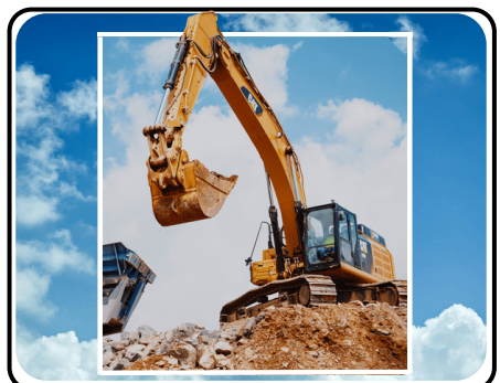
TSR EXCAVATING & SNOW REMOVAL (MONTROSE, SD)
