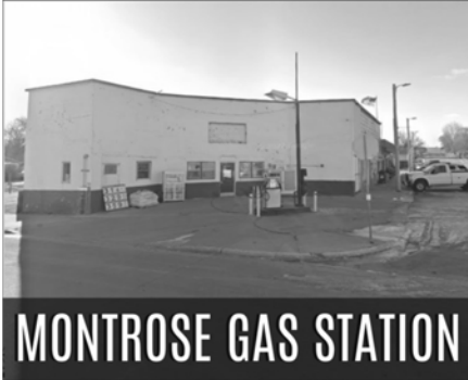
Montrose Gas Station 101 Main Street
